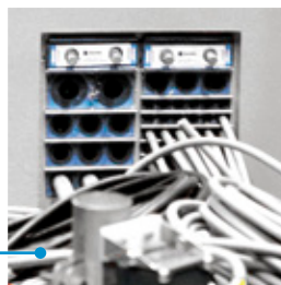
Utility/process areas: Cables to pressure sensors sealed in airtight, fire rated steel frames.
