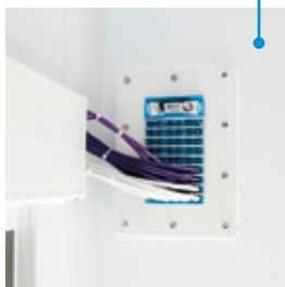
Bio safety laboratory: A powder coated easy-to-clean Roxtec frame sealing a wall transit.
